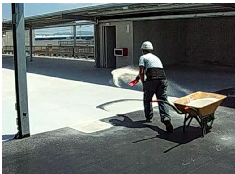
Broadcasting of oven-dry Silica Sand (cornsize 0,1-0,3mm) on the still wet MARISEAL 250 until full saturation.
