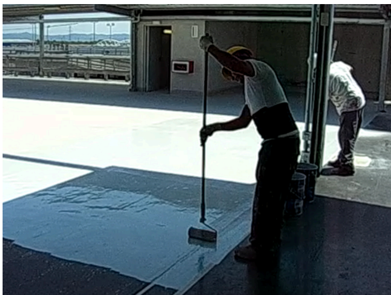
Application of the MARISEAL 250 on the main surface to be waterproofed.
