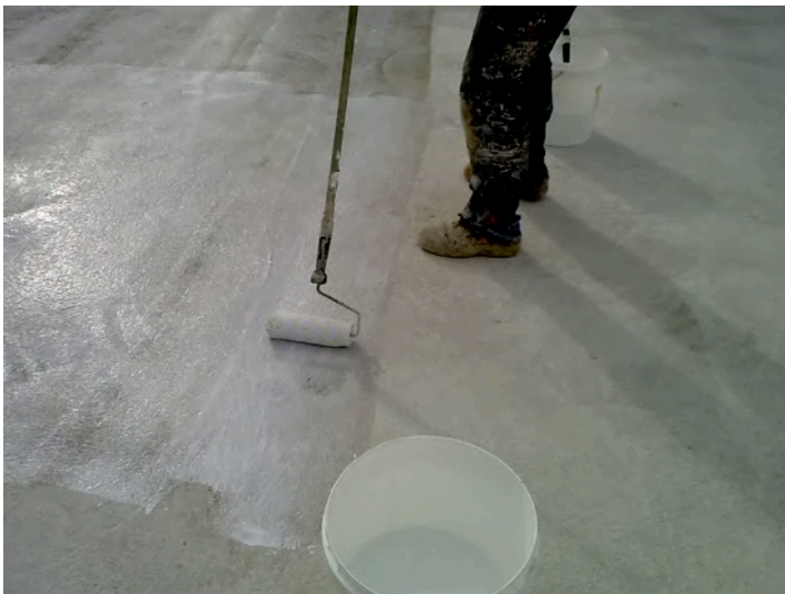
Apply the suitable MARISEAL primer by roller
