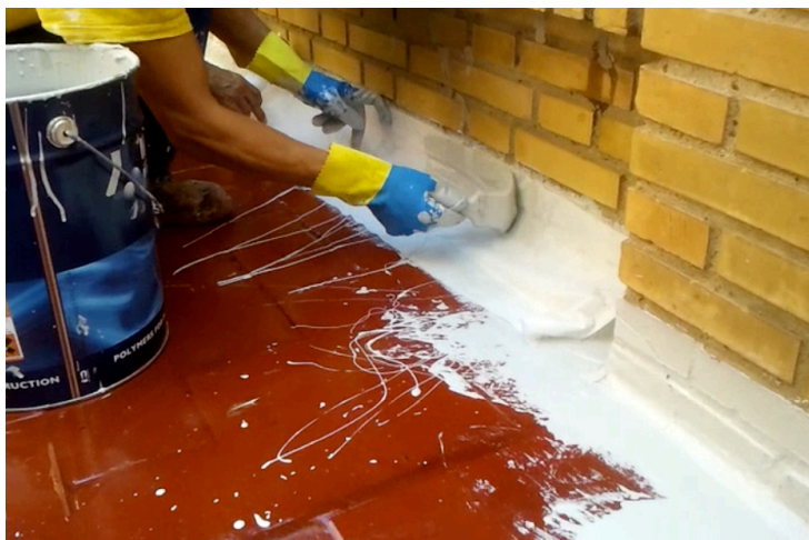
Wall-floor connection (flashing) waterproofing by reinforcing the MARISEAL 250 with MARISEAL FABRIC
