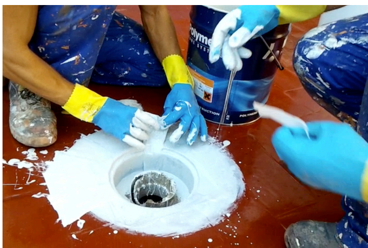
Waterspout (siphon) waterproofing by reinforcing the MARISEAL 250 with MARISEAL FABRIC
